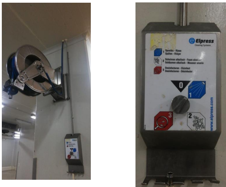
Figure 1-12 Automated cleaning system at the Hawa Chicken Facility
